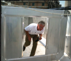
Walkthrough Center Gate/Baffle
